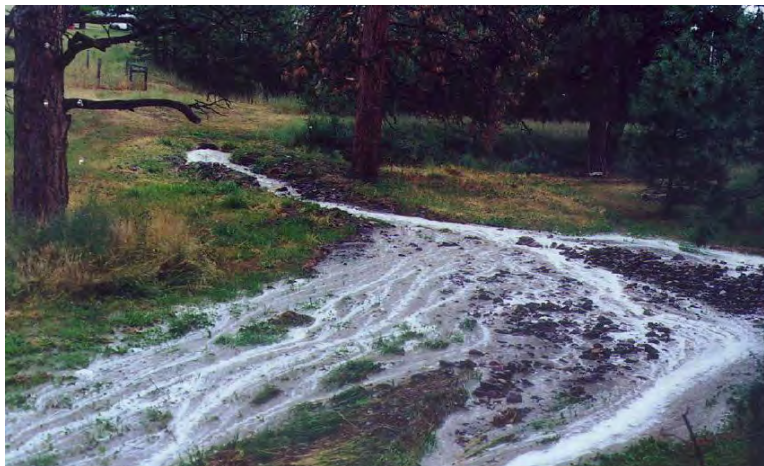
Figure 4.3.11-1 Erosion deposition after runoff event
