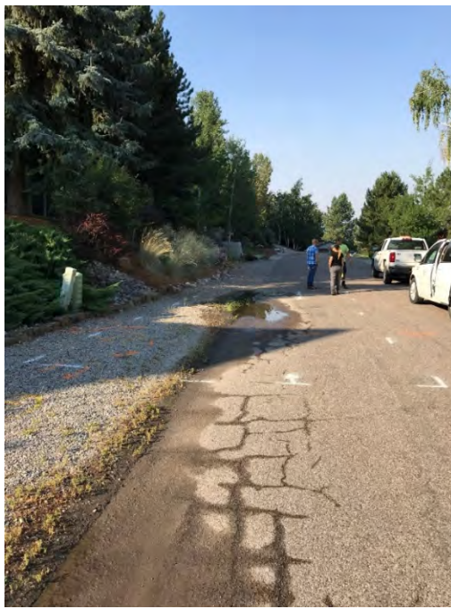
Figure 4.3.2-1 Rosewood Court filled in drainage ditch
