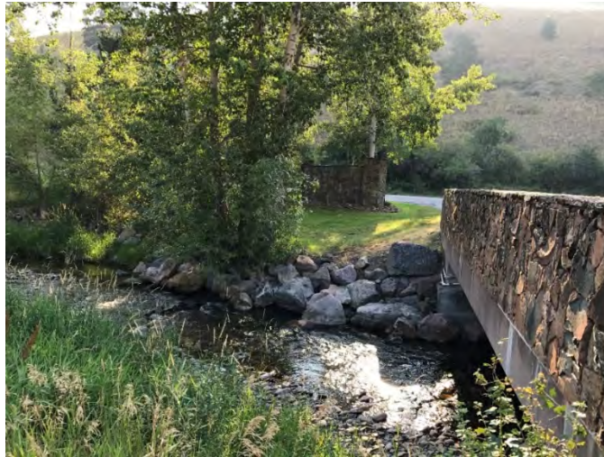
Figure 4.3.1-1 Grant Creek looking downstream from Prospect Dr. Bridge
