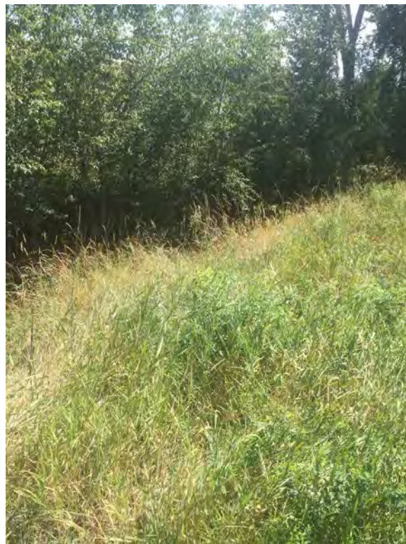
Figure 4.3.1-2 Grant Creek Levee illustrating dense vegetation
