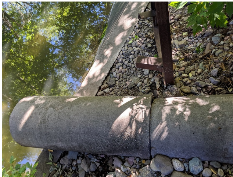
Photo 11. SNA-1519, showing no seal between pipe sections (September 4, 2019)
