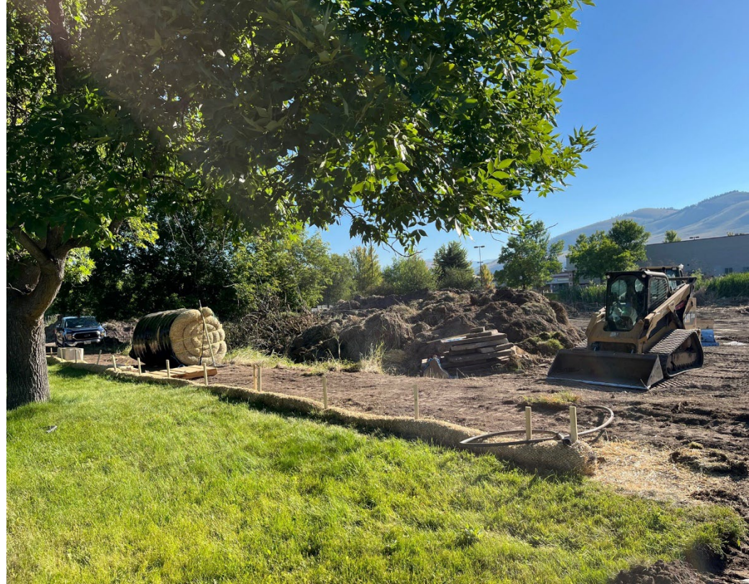
Construction project at Cattail Corner to remove accumulated sediment and debris and improve stormwater storage
