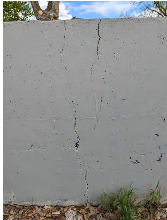
Photo 10. Cracking (Clark Fork Area III Station 20+00)
