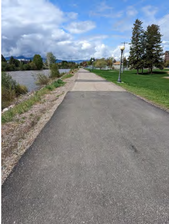
Photo 3. New pavement fixing previous asphalt depression (Clark Fork Area III Station 37+50)
