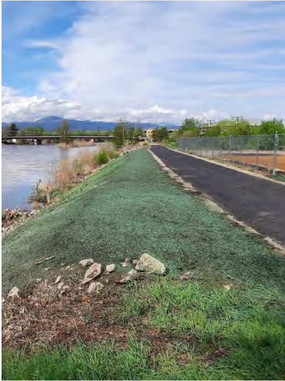
Photo 15. Recent seeding efforts on levee slope (Clark Fork Area V Station 12+00)
