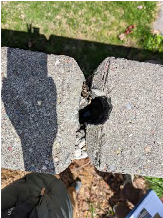
Photo 7. Floodwall displacement (Clark Fork Area III Station 26+00)
