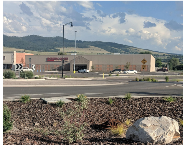
Bioswale with dry well at Southgate Mall
