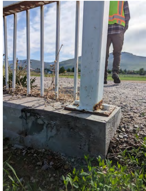
Photo 31. Patched concrete crack at western boundary of Western Detention Basin
