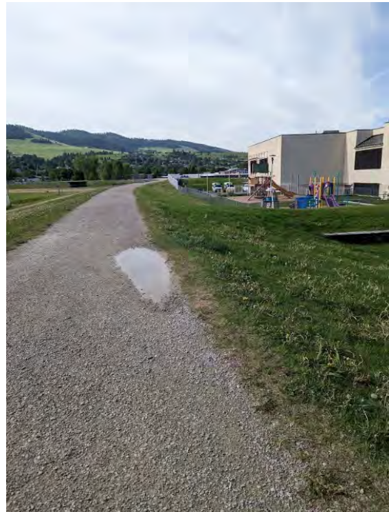
Photo 35. Minor depression along western walking trail for Western Detention Basin
