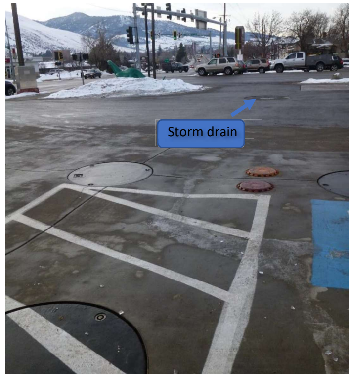
Dry well located directly downgradient from tank fueling area. Another storm drain along the road curb is also downgradient and leads to an outfall on Rattlesnake Cr.
