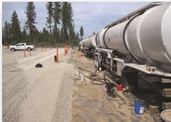
Temporary fueling site with liners under both storage and offload/onload lane (Note black inspection ports along lane). Photo credit: Panhandle Health District.
