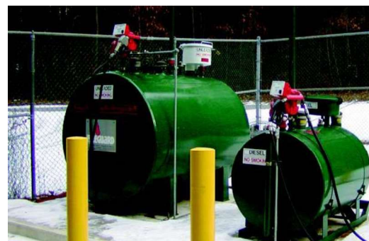
These ASTs are mounted on level impermeable ground with barriers to prevent vehicle collisions. Photo credit: Purdue Extension.
