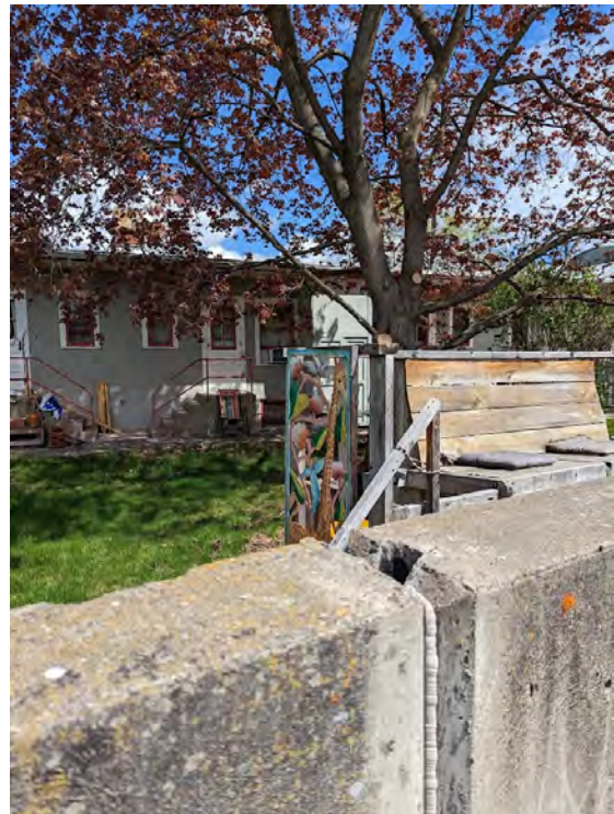
Photo 8. Top view of floodwall displacement (Clark Fork Area III Station 26+00)
