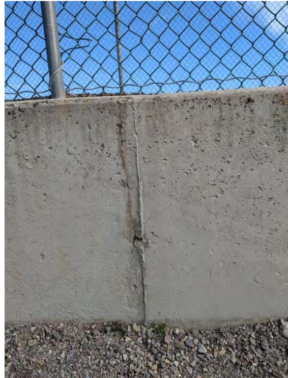
Photo 37. Patched concrete wall on Western Detention Basin
