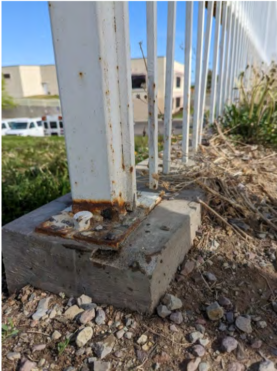
Photo 32. Patched concrete crack at western boundary of Western Detention Basin
