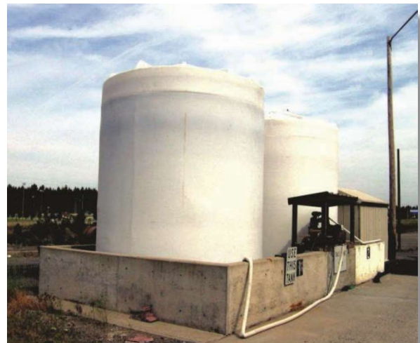
Concrete box containment. Photo credit: Panhandle Health District
