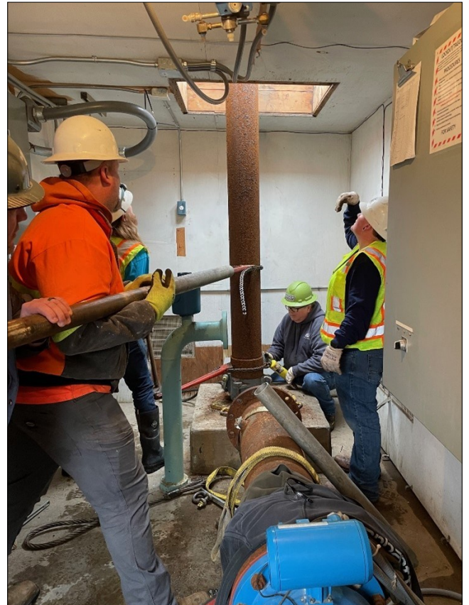
Missoula Water staff and contractor crew combine forces to remove lineshaft turbine pump from water well site.
