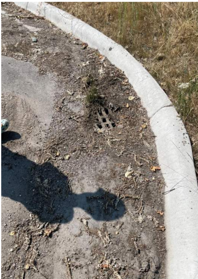
Figure 3-24: Drywell inlet and evidence of ponding at Fox Farm Rd. and Creek Crossing Rd, 2024
