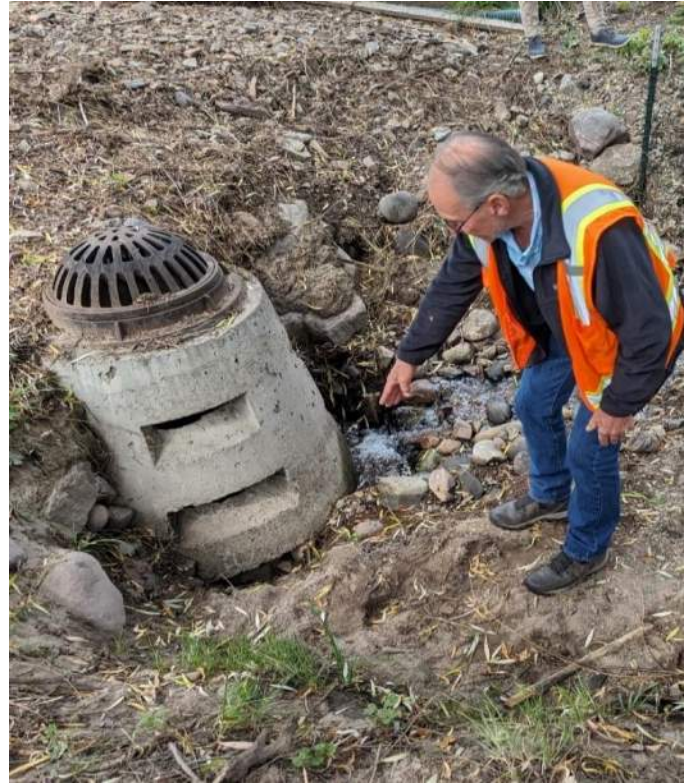
Figure 3-2. Previously installed beehive inlet structure along Continental Way, 2023.
