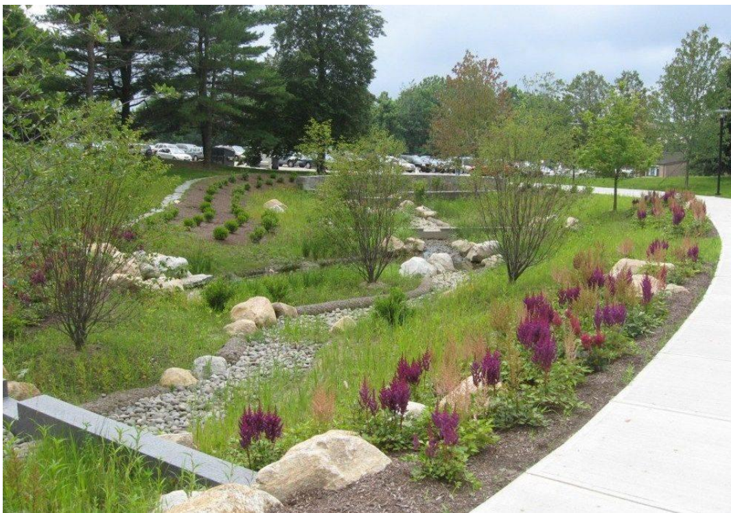
Figure 3-22: Example of a landscaped bioretention area with low flow channel.
