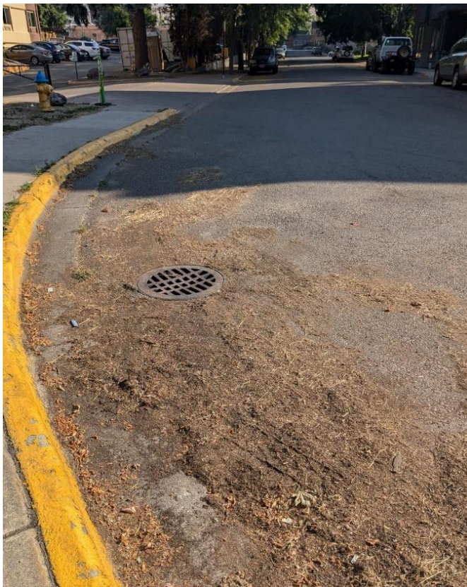
Figure 3-20. Gravity main inlet and evidence of ponding upgradient of Clay Street outfall, 2024.
