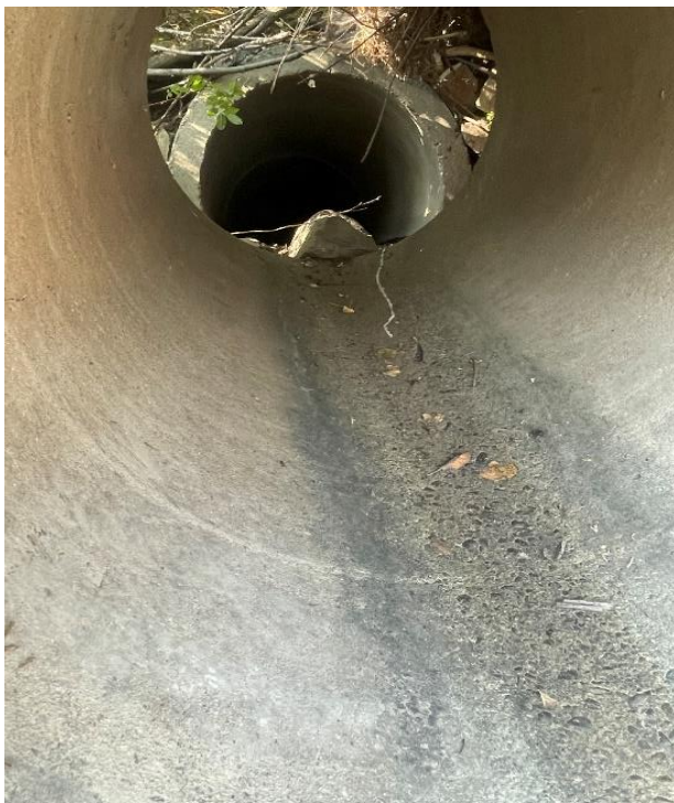
Figure 3-8: Looking inside the damaged outfall structure. 2024.
