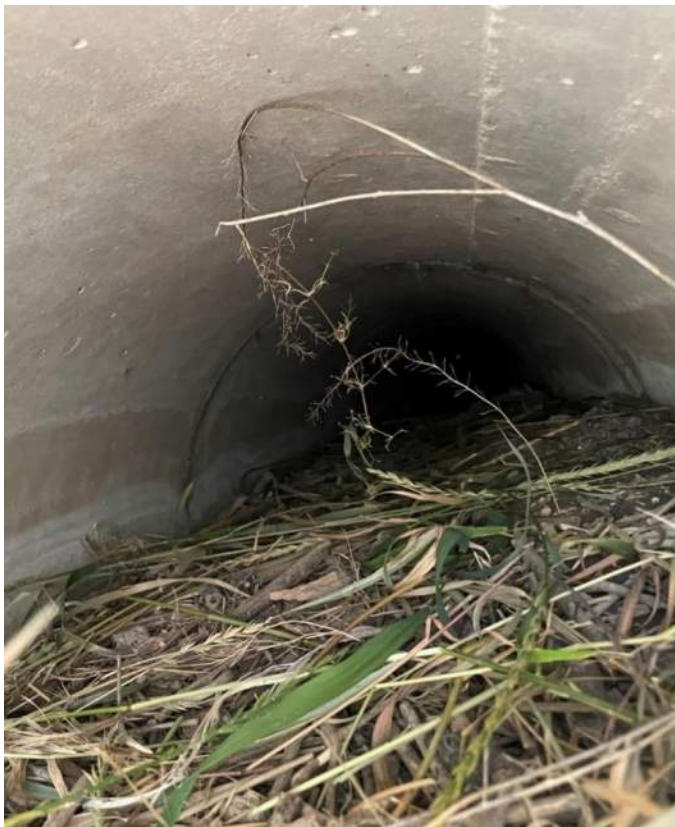
Figure 3-30. Clogged culvert under railroad upgradient of the outfall, 2024.
