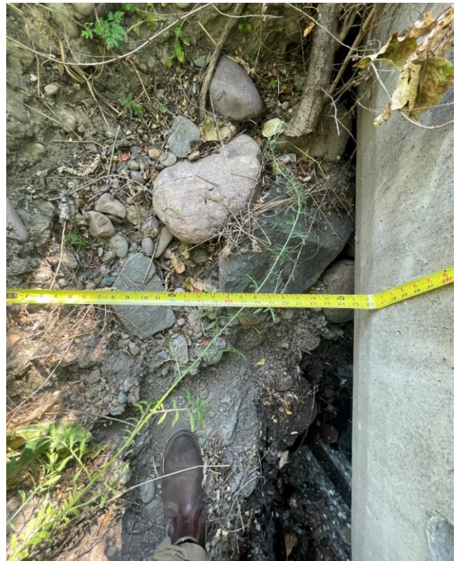
Figure 3-16. Erosion around Fox Site outfall pipe, 2024.
