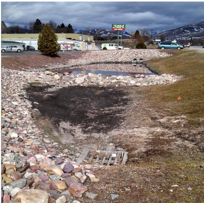
Figure 3-18. Roadside sedimentation pond, partially full, 2015.
