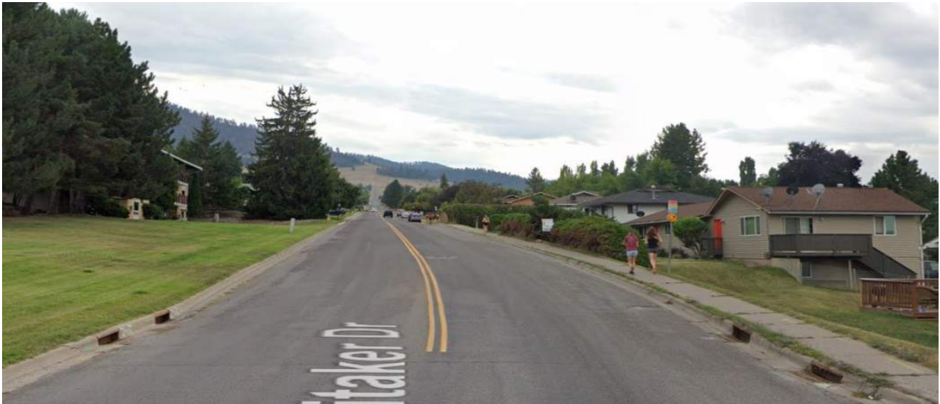
Figure 1-3: Whitaker Drive inlets intercept upgradient runoff
