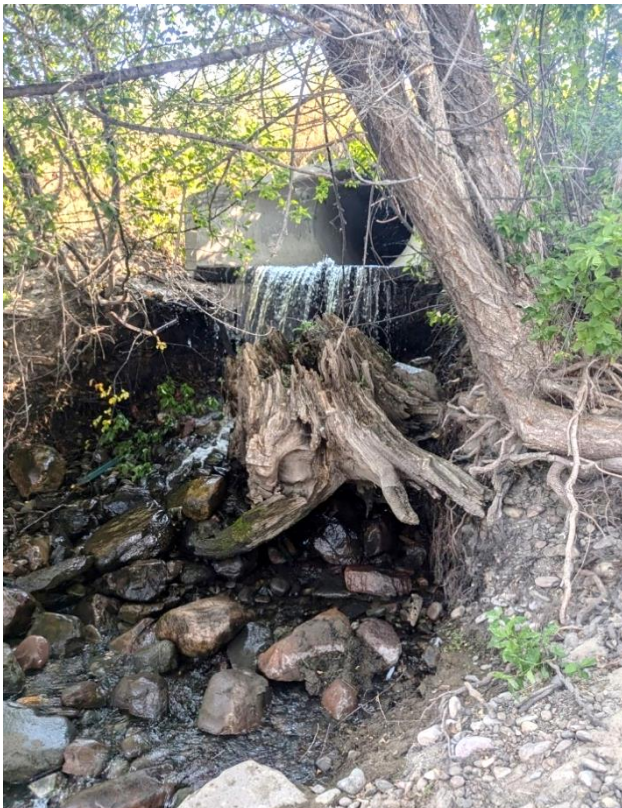
Figure 3-15. Erosion and dry weather flow Fox Site outfall, 2024.
