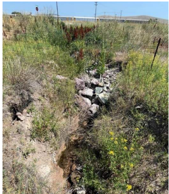
Figure 3-4: Erosion and installed riprap near the Whippoorwill outfall, 2024.
