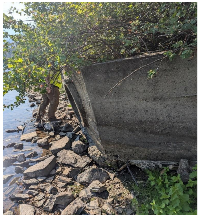
Figure 3-7. Damaged outfall structure. 2024.
