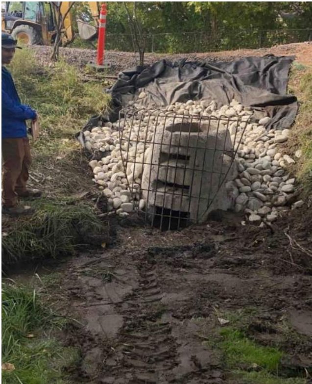
Figure 3-1. Beehive inlet structure being installed along Rimrock Way, 2023.
